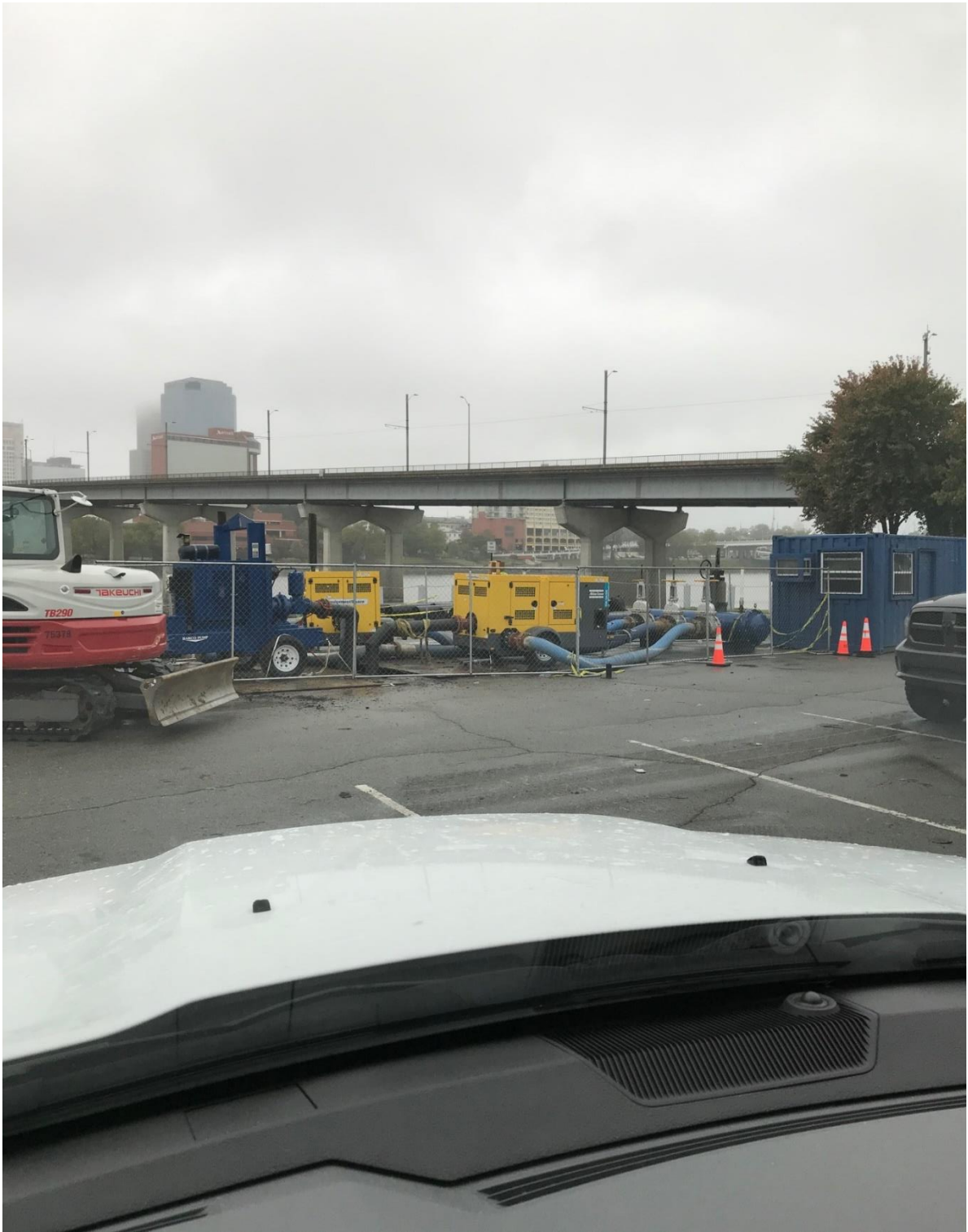
Upper Riverside Interceptor CIPP – October 27, 2020
