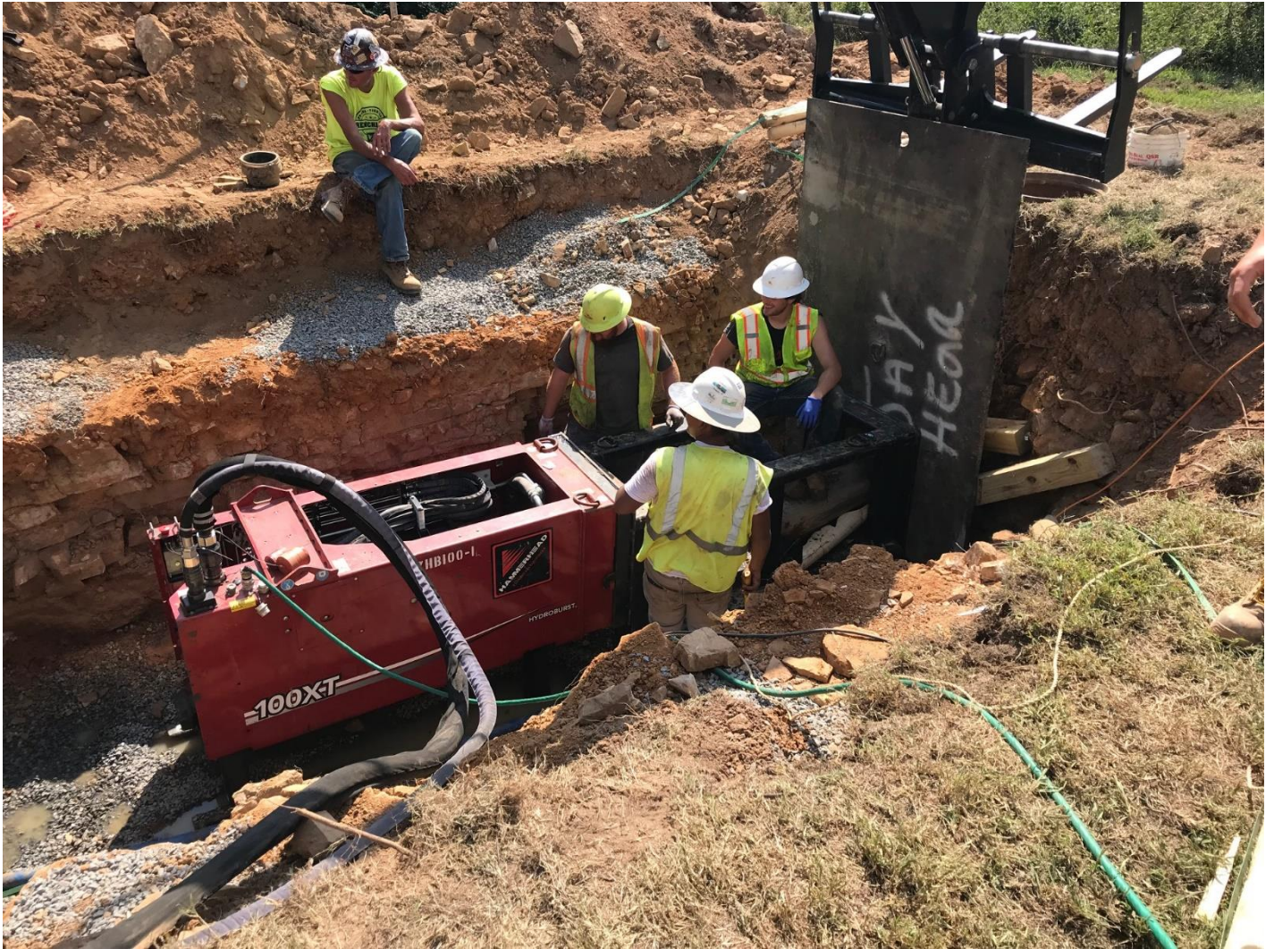
South Levy Pipe Bursting – September 18, 2019
