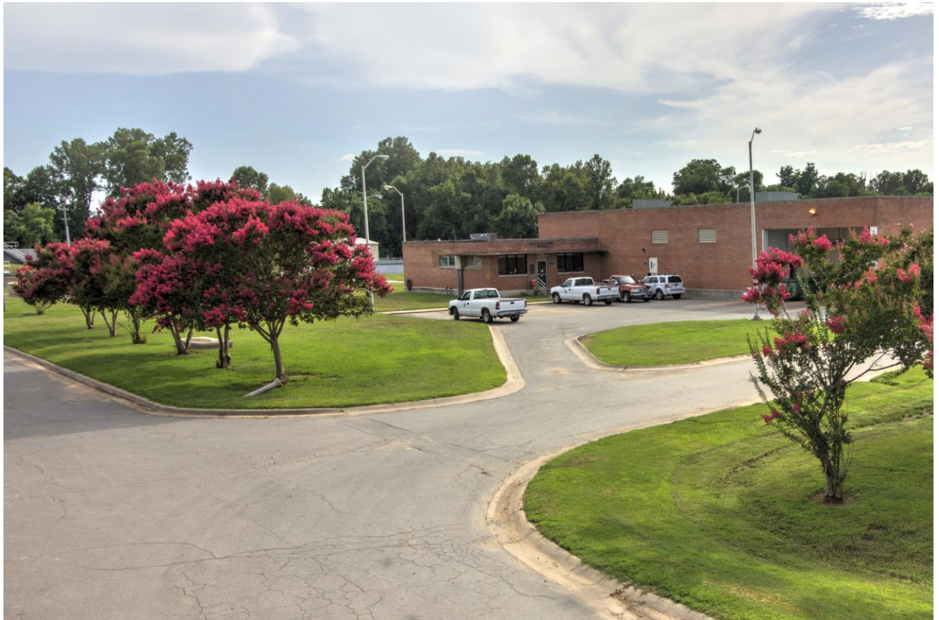
Operations Building at NLRW Faulkner Lake WRF – July 2015
